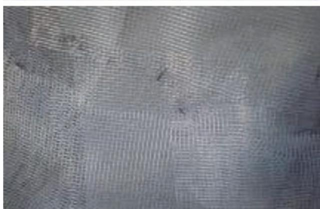
Figure 6. Second covering using wire mesh properly secured and overlapped.
