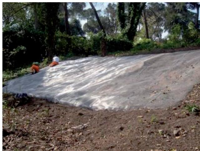
Figure 2. Technicians laying down wire mesh.
