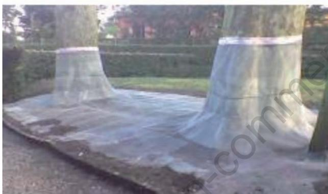
Figure 8. Wire mesh covering trunks and soil.
